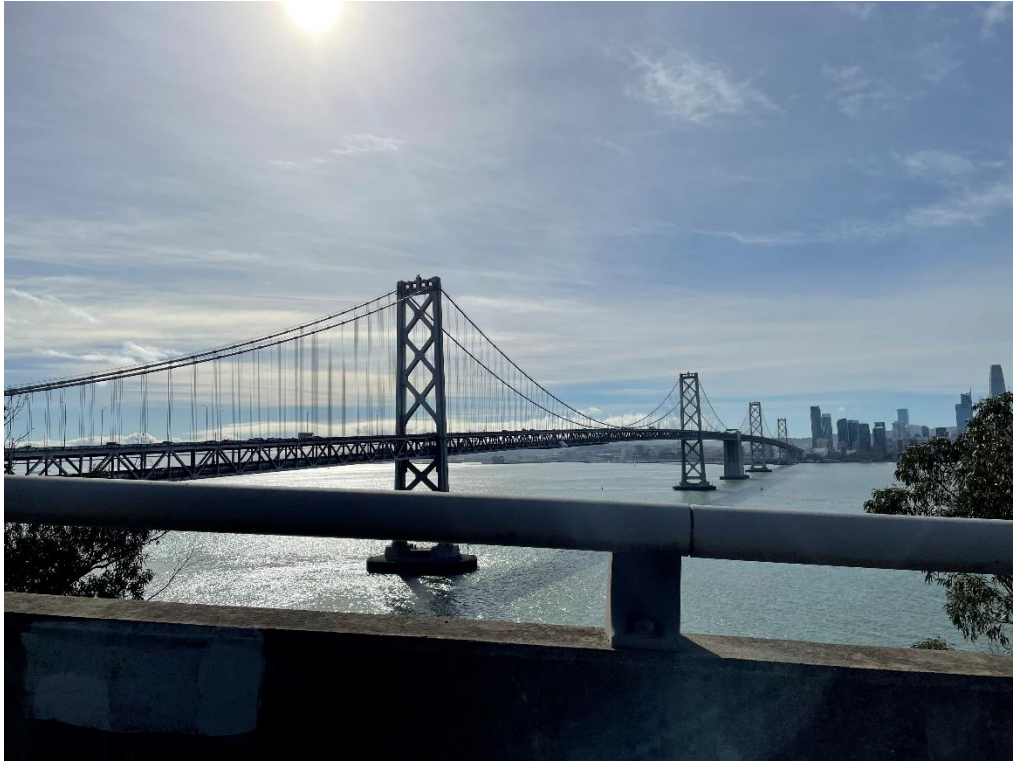
Photo 3: View of the Bay Bridge looking west from Yerba Buena Island, towards the San Francisco shoreline.
