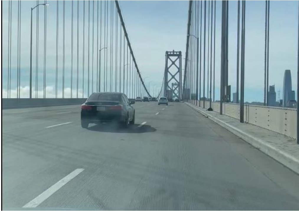
Photo 5: View of suspension cables of the Bay Bridge looking west, toward the San Francisco shoreline, from upper deck of the Bay Bridge.
