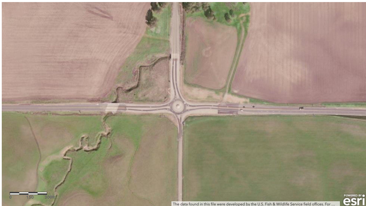
Figure 32. Aerial photograph of completed roundabout at intersection of State Route 12 and State Route 113.
