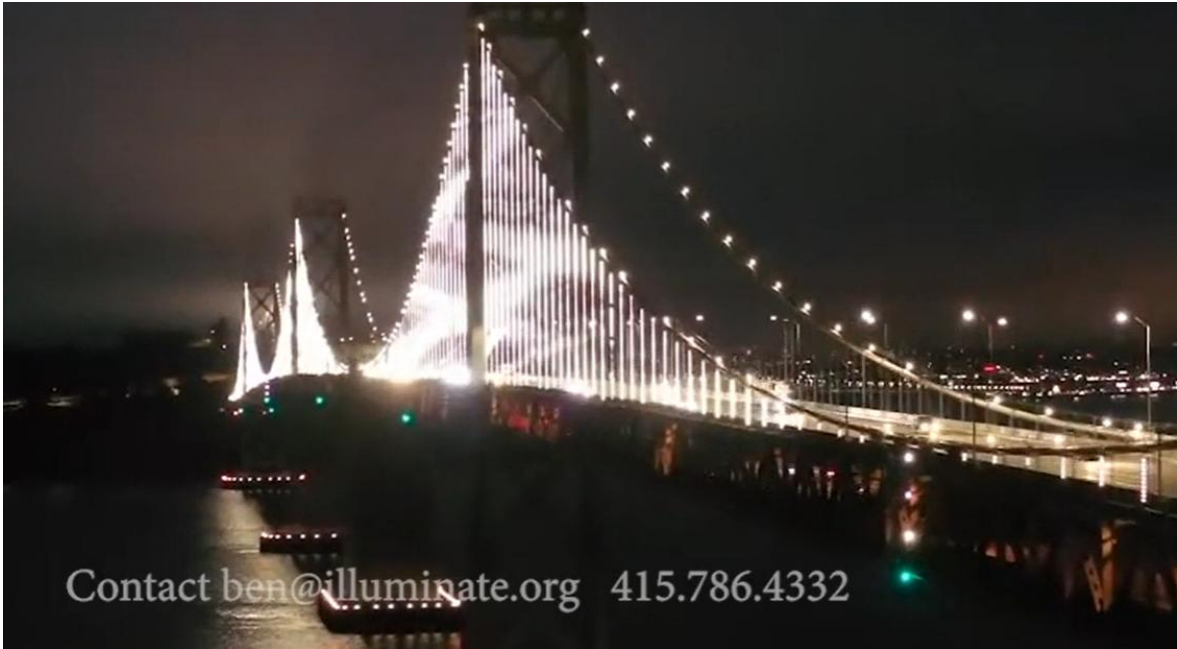
Figure 1 - Glare and Light Pollution from Bay Lights
